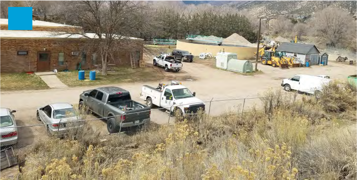
Former Wastewater Treatment Plan prior to demolition.
