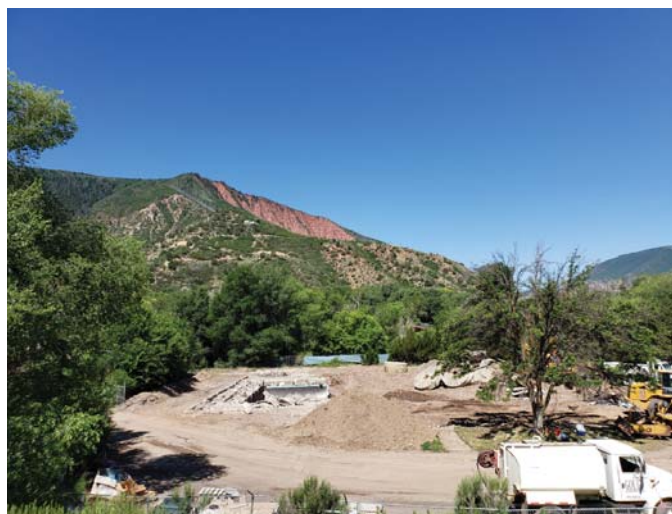
Figure B2: WWTP demolition progress (July 2019).
