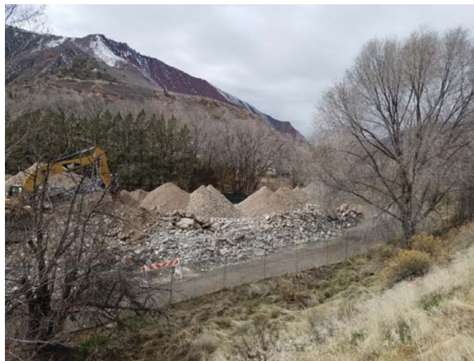
Figure B1: WWTP demolition progress (March 2018).
