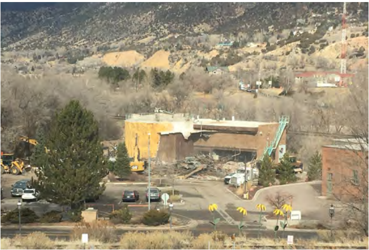
Portions of the Former Wastewater Treatment Plan are being demolished.
