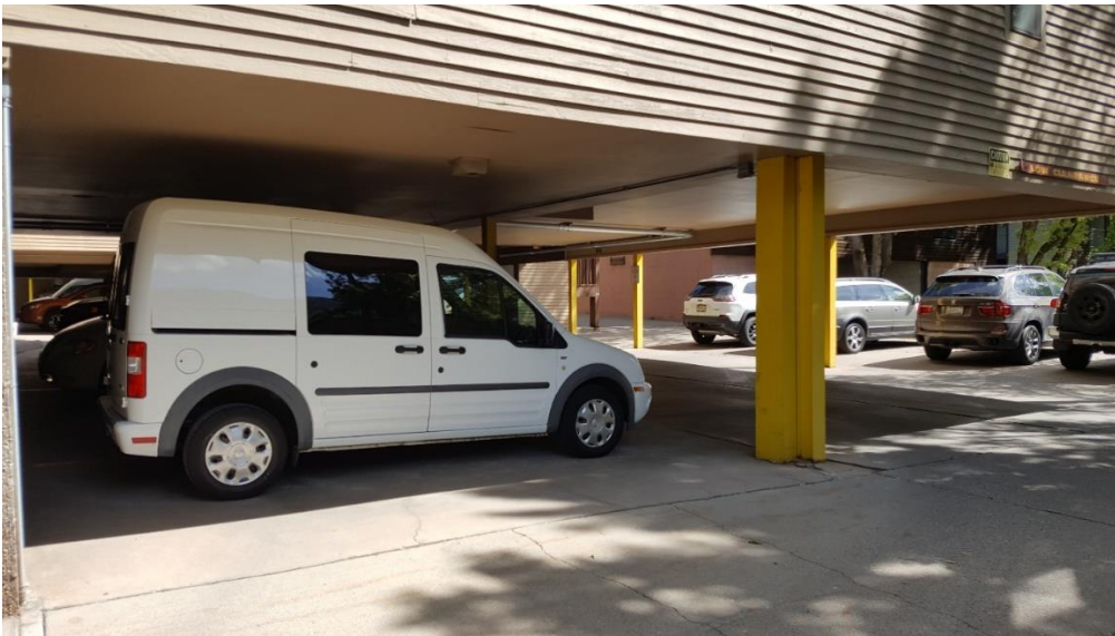
Looking southeast from existing driveway at 410 20 th Street, showing tuck under parking
