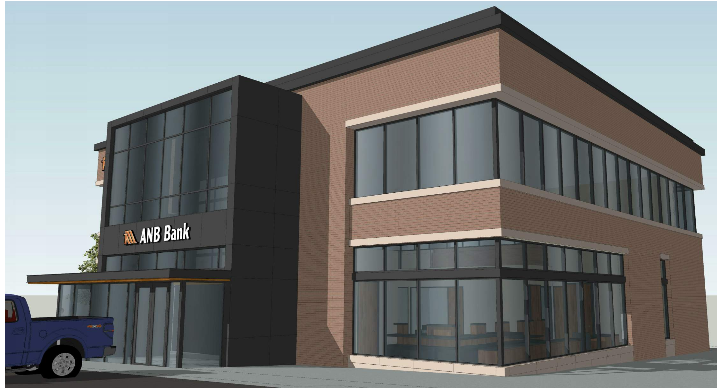
VIEW OF BUILDING FROM ALLEY ACCESS
