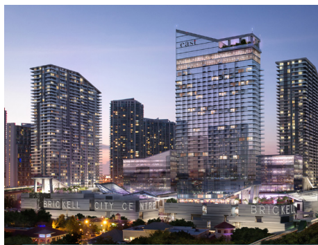
Brickell City Centre Miami, FL
