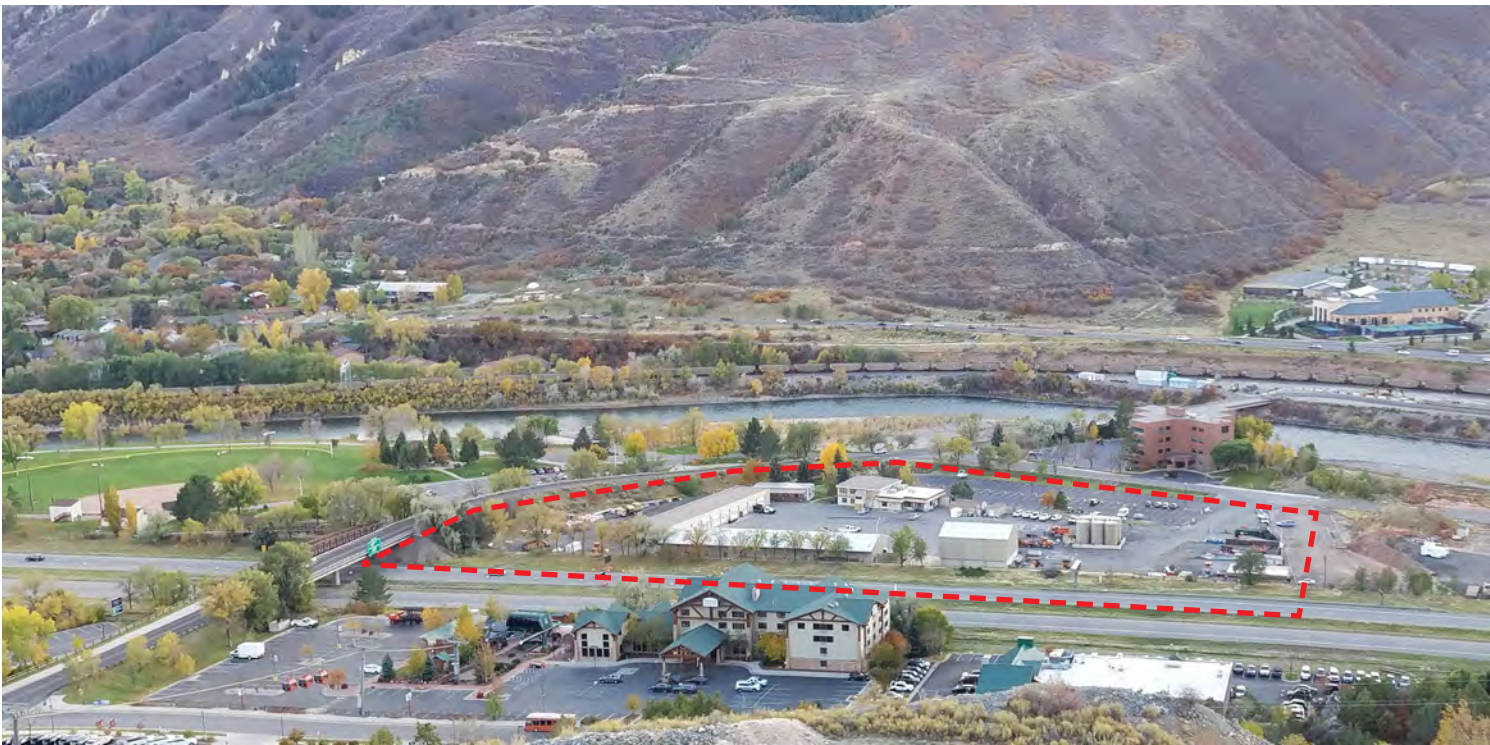
The CDOT Engineering & Maintenance Center
