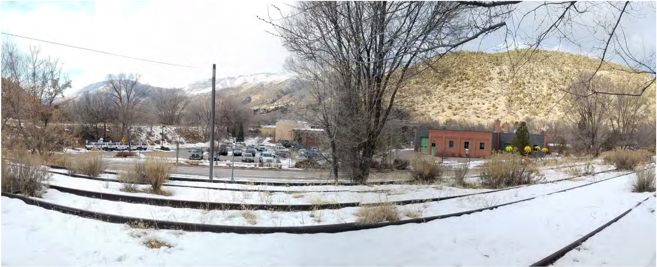
View of the Former Wastewater Treatment Plant. Note building to the right is the new active pump station.
