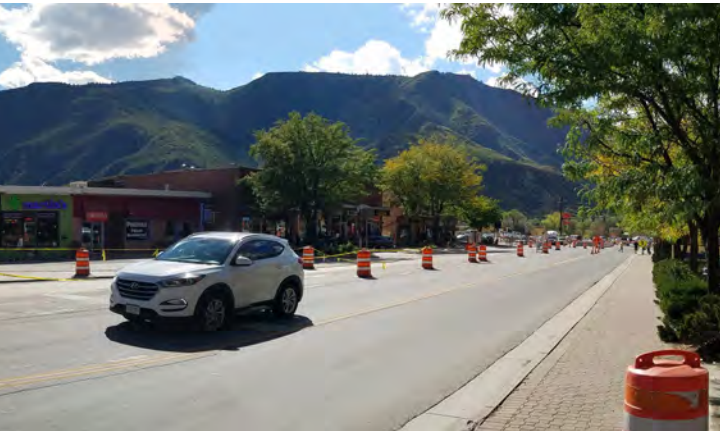
6th Street under construction
