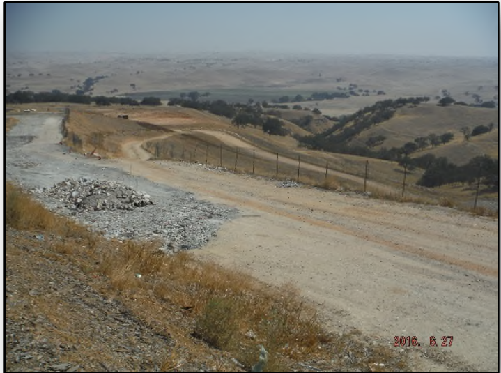
Unprocessed Concrete Used for Access Road
