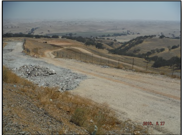
Unprocessed Concrete Used for Access Road
